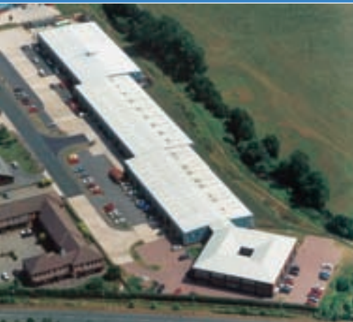
Tiverton UK – Head office at main manufacturing site
